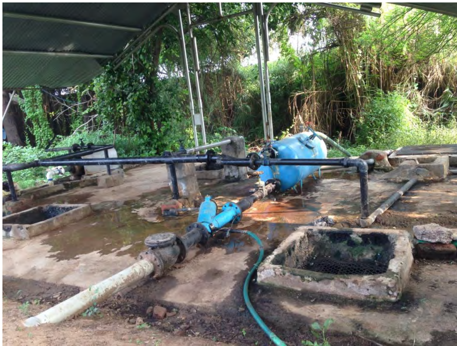
Silicon sand filter at DA-IICT
