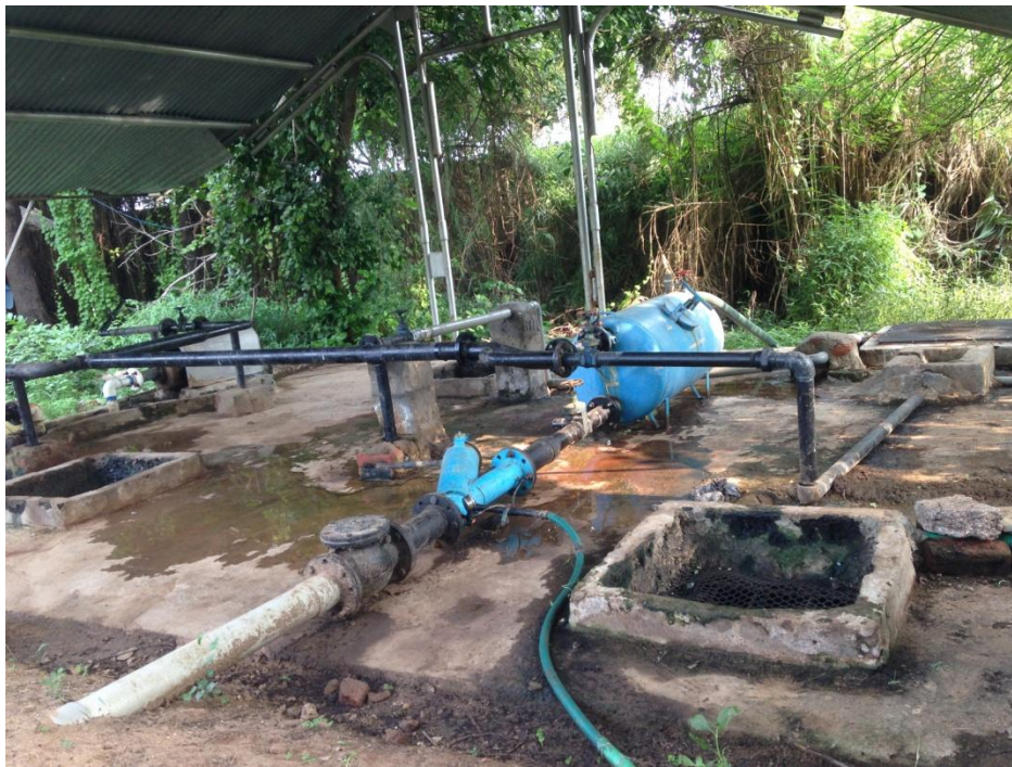
Silicon sand filter at DA-IICT
