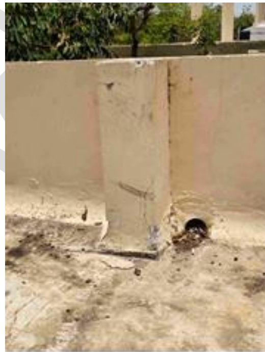
Accumulation of Water and dust near OHWT
