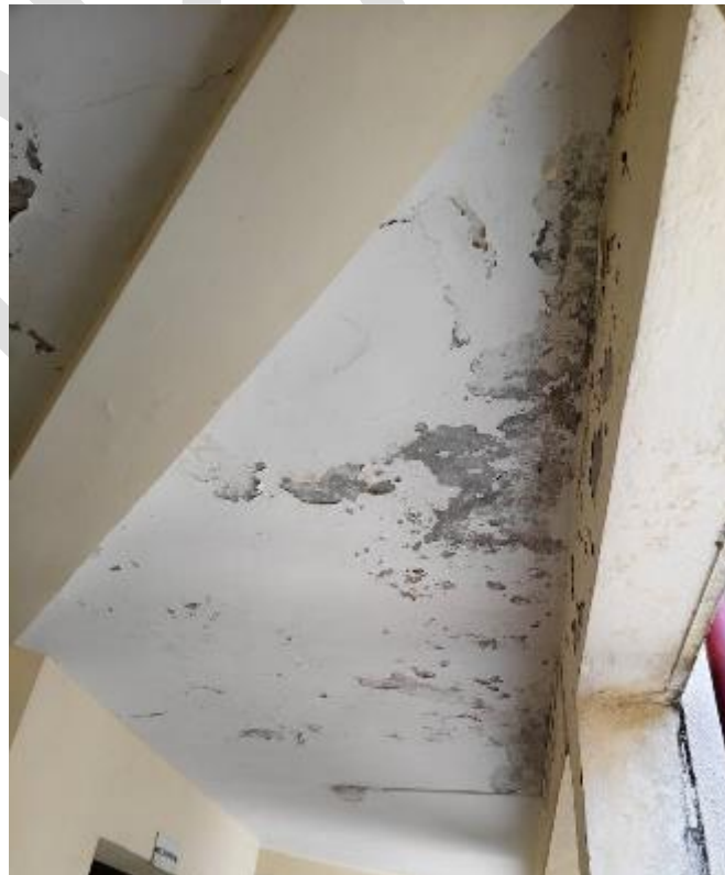
Slab concrete spalling off due to corrosion of steel and wall cracks at wall Beam junction.
