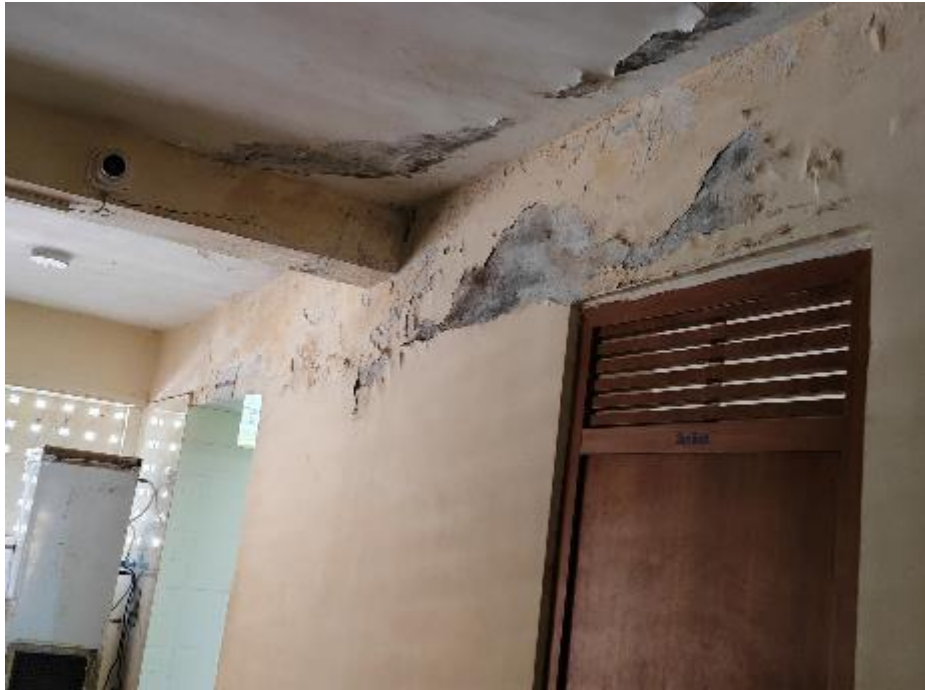
Leakage near Toilet block
