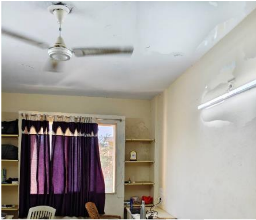
Slab concrete spalling off due to corrosion of steel and wall cracks at wall Beam junction.
