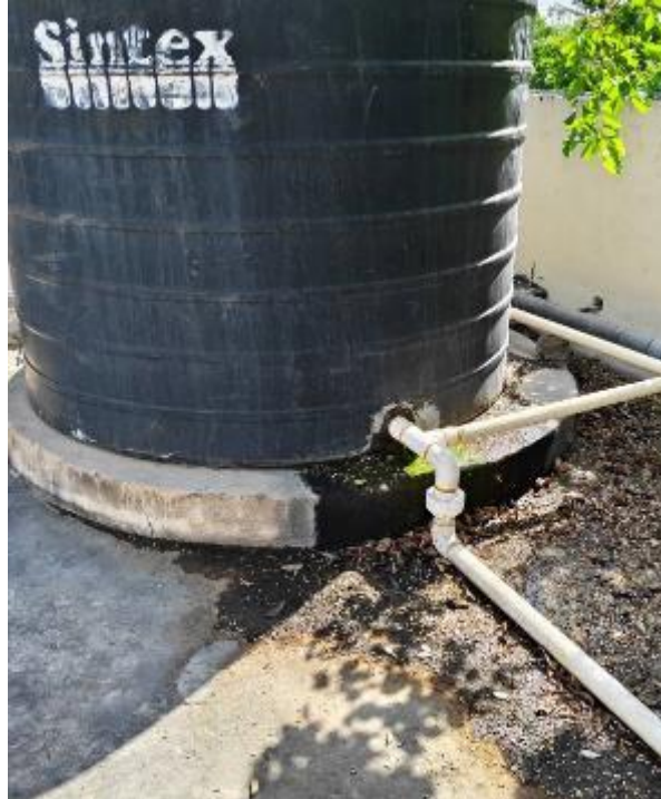
Accumulation of Water and dust near OHWT
