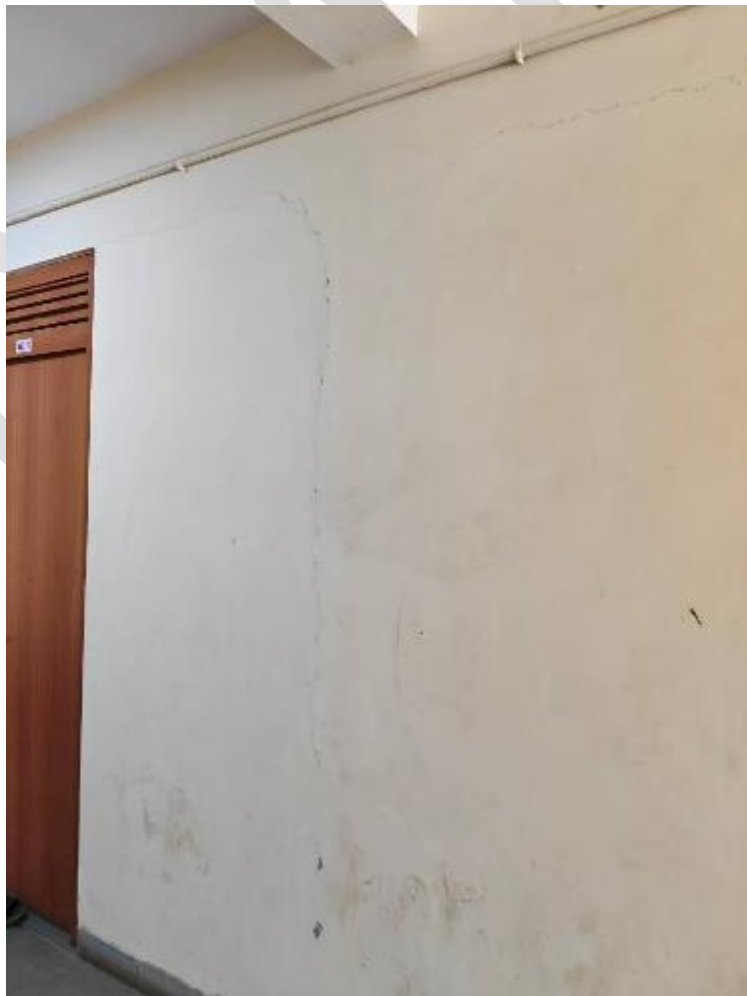
Cracks at beam Bottom Level
