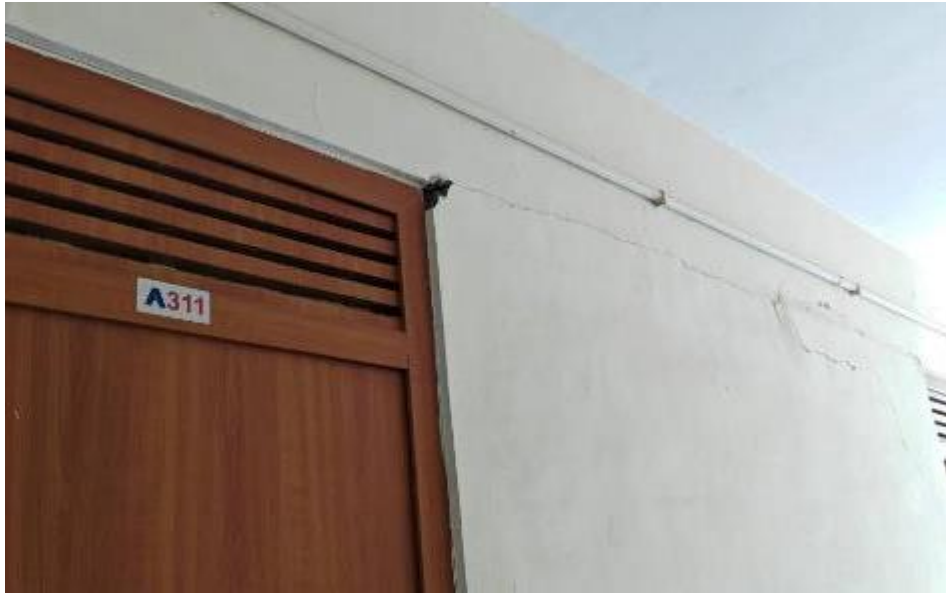
Cracks at beam Bottom Level
